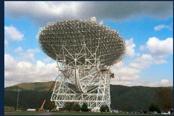
The receiver has diameter about 100m. Radio waves of wavelengths from 30 cm down are studied. Angular resolution around 0.15°.
