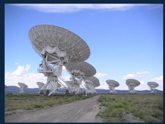
The effective D is the length of the line of telescopes.
